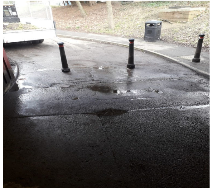
Woolborough Lane: Before cleaning
