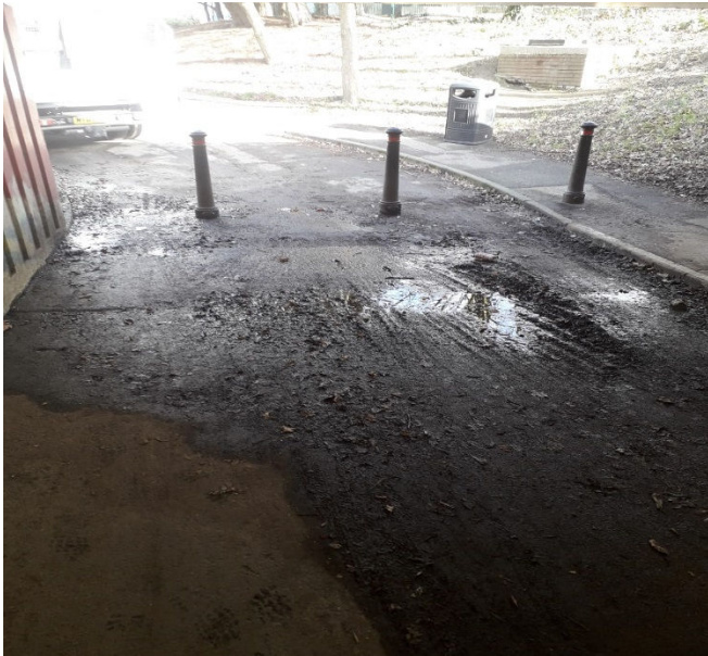
Woolborough Lane: Before cleaning
