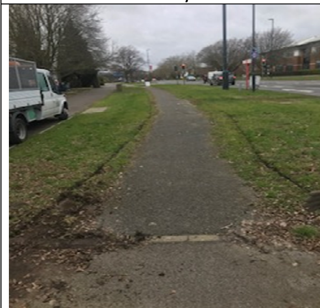
Edging along Manor Royal Road - Before
