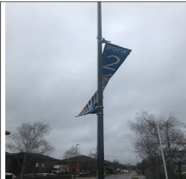
Example of wind damage to a banner
